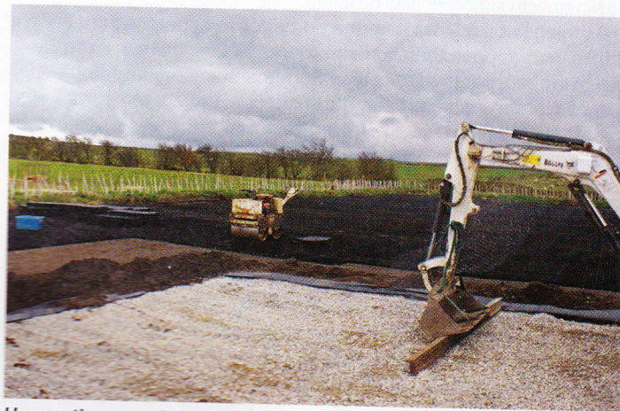
Hexapath car park surface being laid
